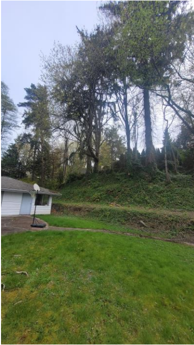
F. “Bench” building pad in foreground. Shelf and then steep easterly slope. Catchment wall will be at toe of slope.
